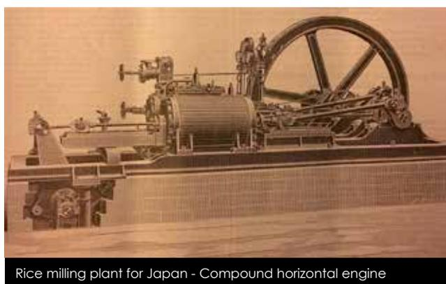
Rice milling plant for Japan - Compound horizontal engine
