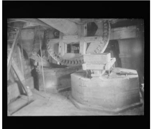
Above: A rare lantern slide from the collection of Ronald Clarke, a well-known author of books on traction engines. It shows the interior of an unidentified East Anglian post mill, with two pairs of millstones located side by side and driven by the tail wheel - an arrangement that can no longer be seen in the UK.
