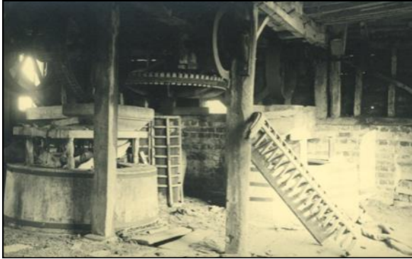
Left: A moody internal view of the millstone floor of an unidentified watermill.
