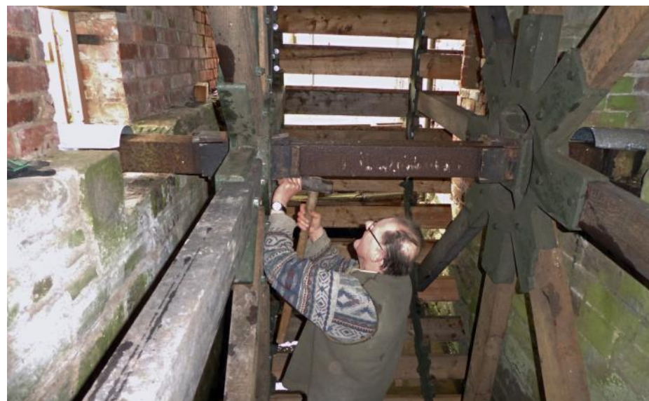
Alan at work tightening wedges in a waterwheel, Court of Noke Mill, Pembridge.
