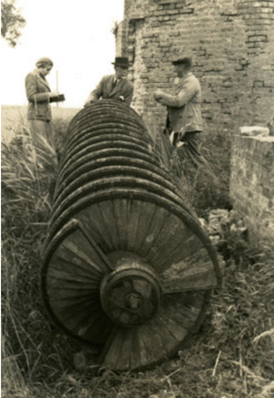
Above: Archimedes' screw, Moulin de l'Hostine at Looberghe (Nord).
