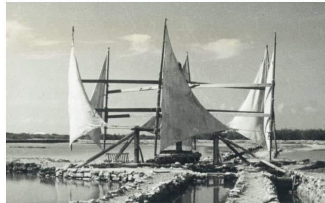
Left: Horizontal windmill at the saltworks, Salt Cay, Turks and Caicos Islands.
