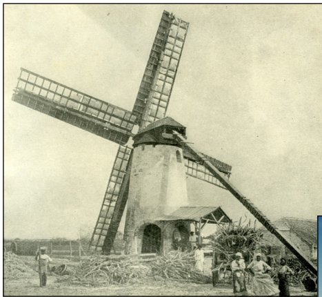
Above: Wind powered sugar cane mill in Barbados showing both male and female workers. Note the extremely long tail pole for turning the cap and sails into the wind.
