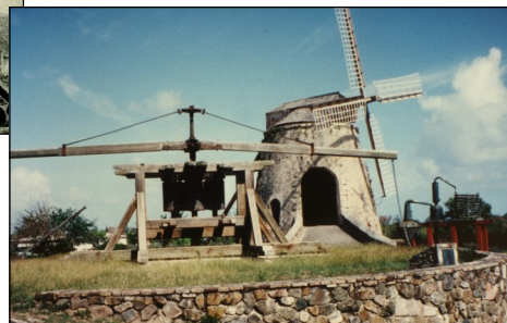
Above: Wind powered sugar cane mill in Barbados showing both male and female workers. Note the extremely long tail pole for turning the cap and sails into the wind.
