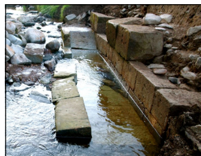
The masonry wheelpit
