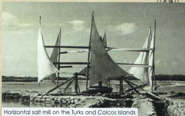
Horizontal salt mill on the Turks and Caicos Islands
