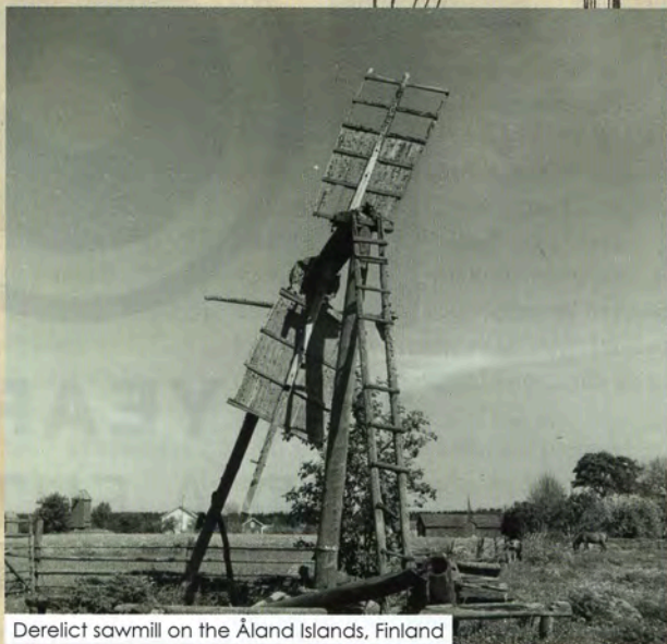
Derelict sawmill on the Åland Islands, Finland
