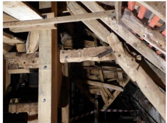
The photo above shows one of the new oak posts supporting the purlins from ground level.
