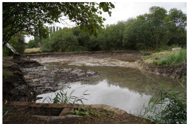
The mill pond after 4500 tonnes of silt had been excavated
