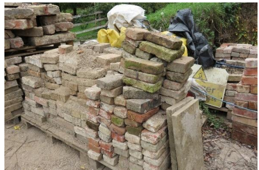
Many of the bricks being used to clad the concrete come from the site, the remnants of the 1797 mill and even older buildings
