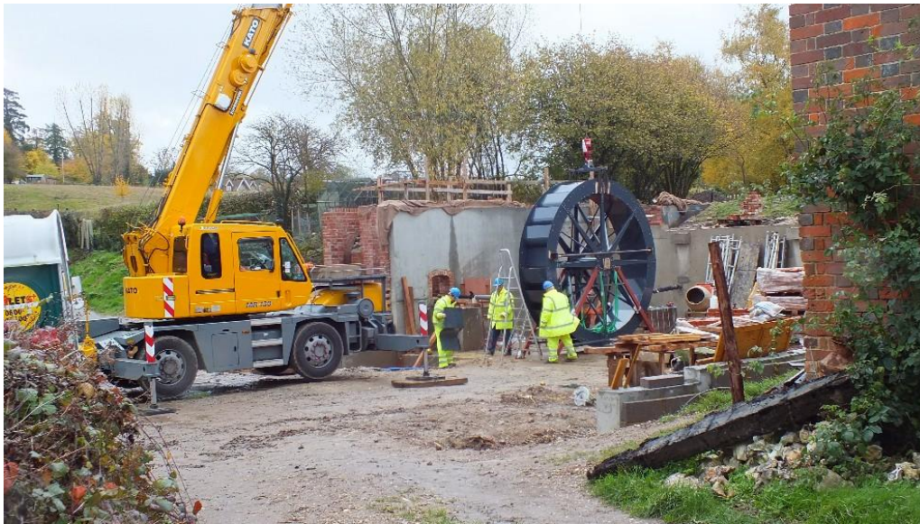
This picture was taken during the process of bolting together the two halves of the wheel; which had to be split to be transported from Cumbria.
