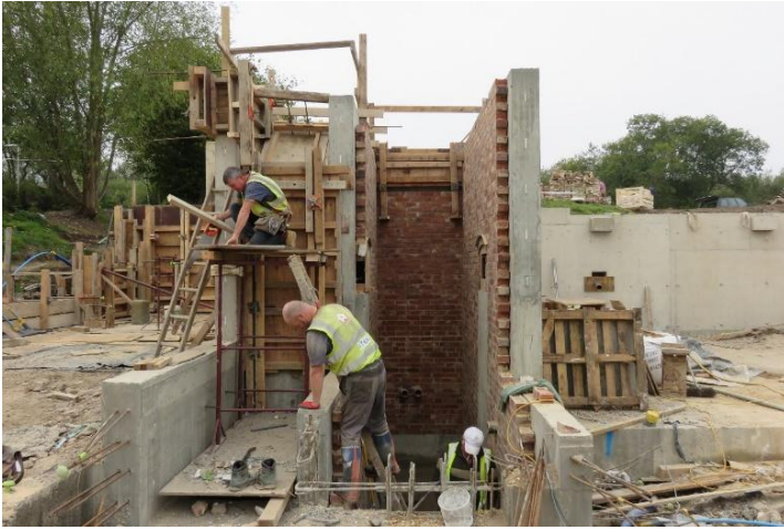
The wheelpit under construction
