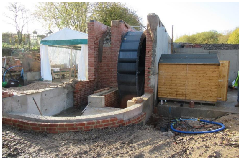
This picture was taken during the process of bolting together the two halves of the wheel; which had to be split to be transported from Cumbria.
