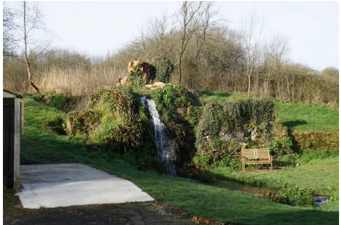
Note the reed bed in the silted mill pond and a woody bole – the remains of a large willow tree that had cracked open the masonry leaf
