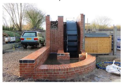
21 November 2018: The wheel was commissioned yesterday and operated at full crack overnight generating Checking it this power. morning though it seems to have shifted along on its axle by about 12cm despite the taper locks that should lock it to the keyway. We have therefore dropped the level down again.
