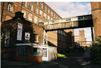
Mutual Mills in Heywood is a group of three cotton mills dating from 1884 to 1914 which were built for the Mutual Spinning Co with additional weaving sheds added in 1927 to 1937. They had steel framing and concrete flat roofs, which meant that conversion to residential apartments was a more proposition. practical Such development by Knight Knox is now under way, as shown in their promotional picture below.
