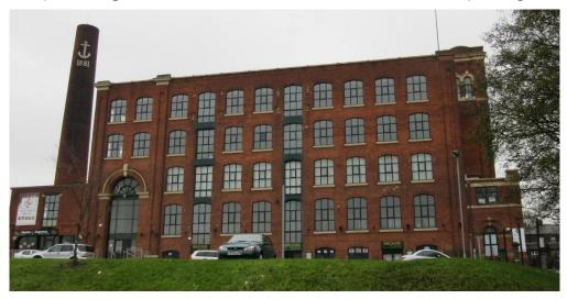
**Anchor Mill** (1881) in Oldham was designed by Joseph Stott. It had an integrated engine house (behind the arched window on the left), an external boiler house next to it, and a
