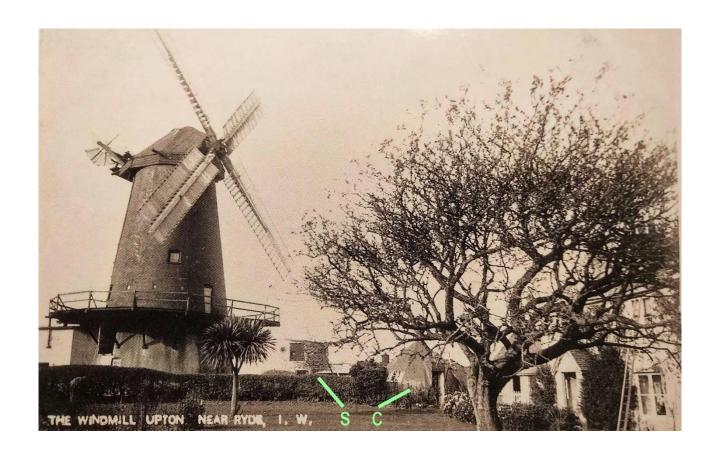
The stage is a wide one, giving easy access to the sails. Visible in the postcard 'front' view on the next page, just below door height at stage level, are what look like 3 equidistant holes, which I think are the sawn off timbers to which the endless chain that turned the cap into the wind could be attached to stop it swinging about. Once hand-winding was replaced by the fantail they became redundant. These were a feature very common on Anglesey windmills and would encircle the tower.
