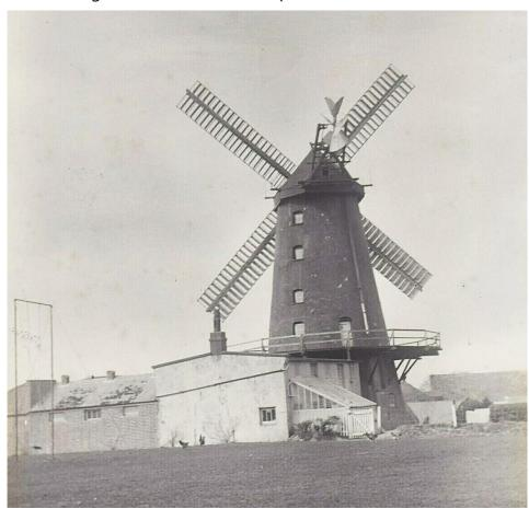
At the rear, what looks like a pipe running down the tower must be a wooden chain guide attached to the cap. This is a common feature on a number of mills in the east of the country, particularly Norfolk, and is to steady the striking chain with weight attached that operates the patent sails.
