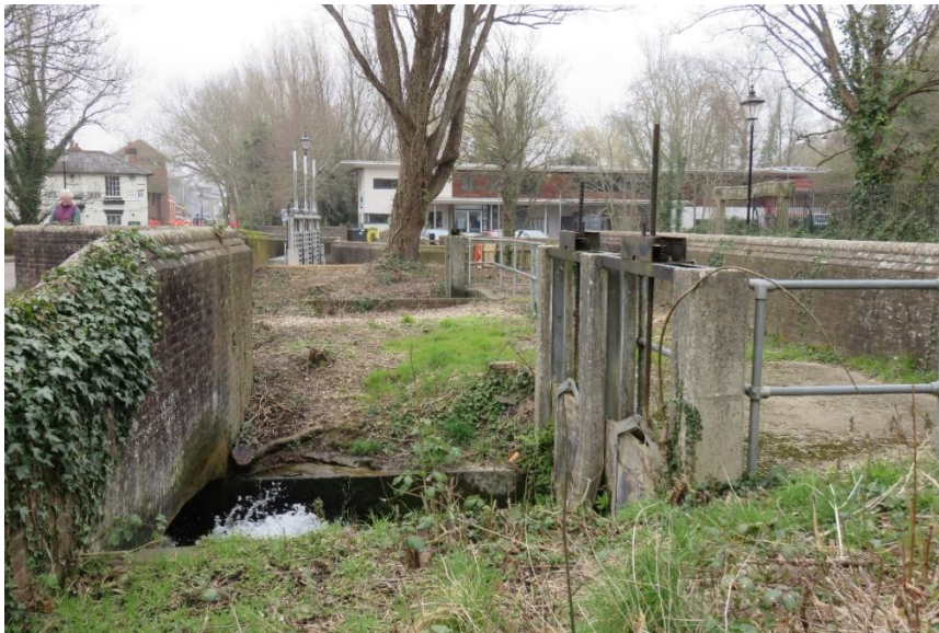
Site of Durngate Mill showing old sluices (foreground) and new sluice 3 in the distance and right
