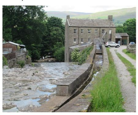
Its water supply still occupies the original stone and timber above-ground launder, which has always been the site's most striking feature when viewed from the road bridge. The wooden section, seen here, must have been mended many times!
