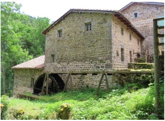
The mill has always relied on water power, with two working horizontal wheels inside (one wood, one and vertical metal) а overshot wheel on an outside wall. There are 4 sluice gates in the mill head which control the water supply from a dam some way upstream.
