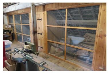
Inside the mill there are several modifications which have been necessary to meet modern food handling requirements. The most noticeable of these changes are the mesh-fronted rodent-proof storage bins for grain.
