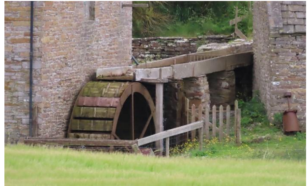
The overshoot waterwheel, about 4.1m diameter, turns at some 12rpm. The water comes from the nearby Boardhouse Loch.
