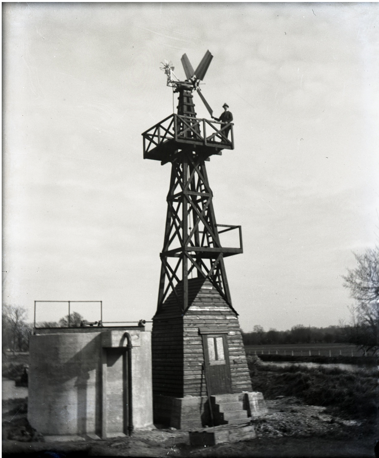
Image 1: Burne Windmill in Thatcham, Berkshire. Taken in the 1920s, this photograph shows a Lancaster Burne wind turbine design, which was sold to private buyers and erected throughout
