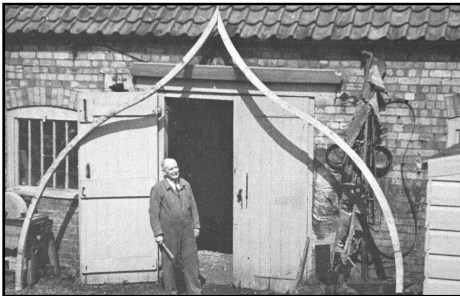
Jack Thompson at the workshop door with a template for the ogee-shaped cap roof of Dobson's Mill at Burgh le Marsh, c1947.
