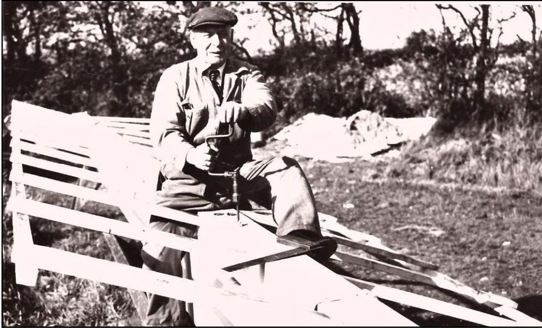
A press shot from 1957 shows Jack Thompson at work on site at Burnham Overy tower mill, Norfolk. He is using a brace and bit to bore a hole for one of the king bolts which fastens the sail whip to its stock.
