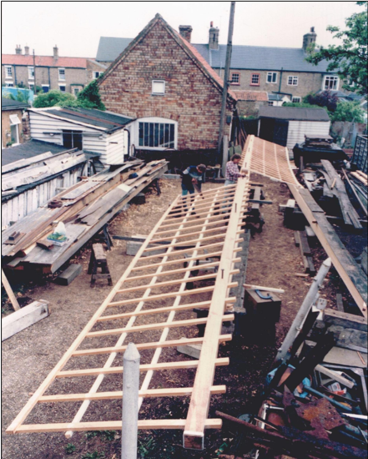
This photograph, dated 1985, shows just how much room a pair of sails occupied when they were laid end to end on their supporting stock. Employees Tim Farnsworth and Denis Moore are shown working on a pair of common sails for Green's Mill, Sneinton, Nottingham. Thompsons completed the restoration of this mill to working order, lifting the sails into place in July 1986. Flour has been milled successfully there ever since.
