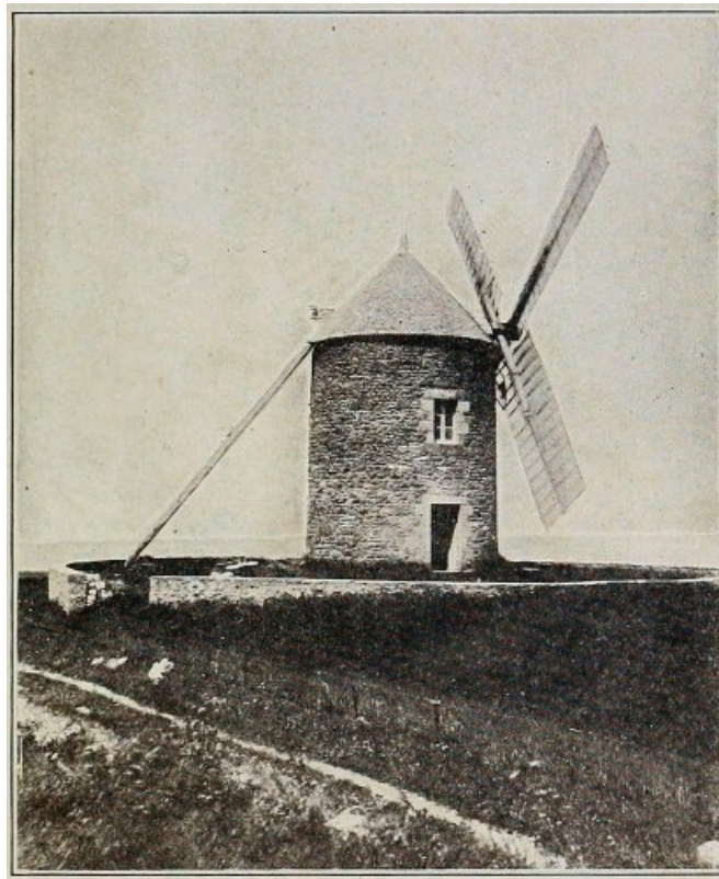
Tower mill and tail beam. St. Lunaire, France.
