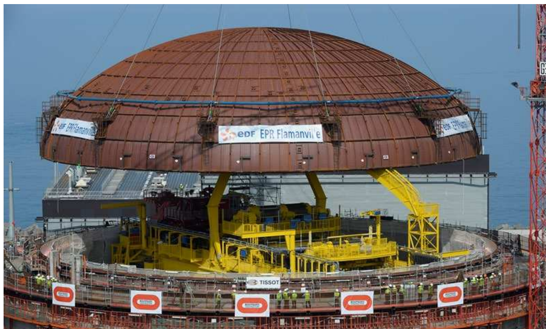
Figure 9.2: Flamanville 3 — dome being lifted into place on reactor building
