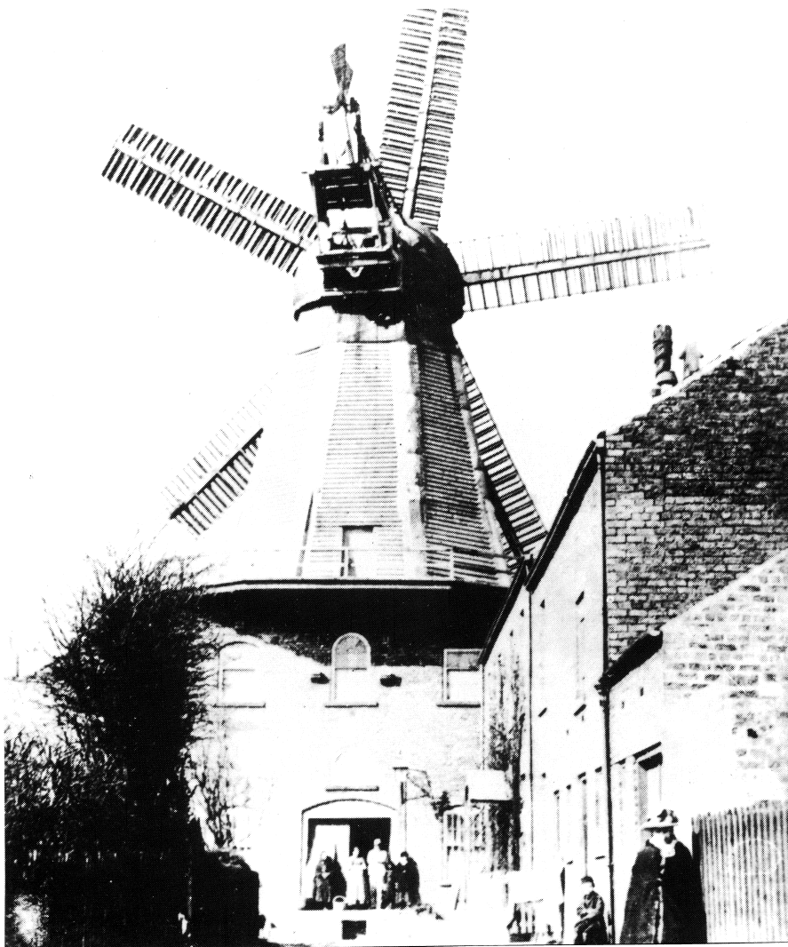
Fig. 1. Chimney Mill, Newcastle-upon-Tyne, in its latter working days (photograph by courtesy of Mr Thomas Falconer)
