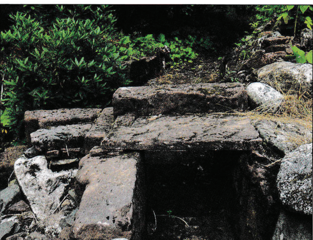
Fig. 10. Shutter board housing controlling flow down mill race.
