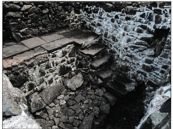
Fig. 7. Platform and base for beams across to riverside wall and flooring. Stone steps to tail race and wheelpit.
