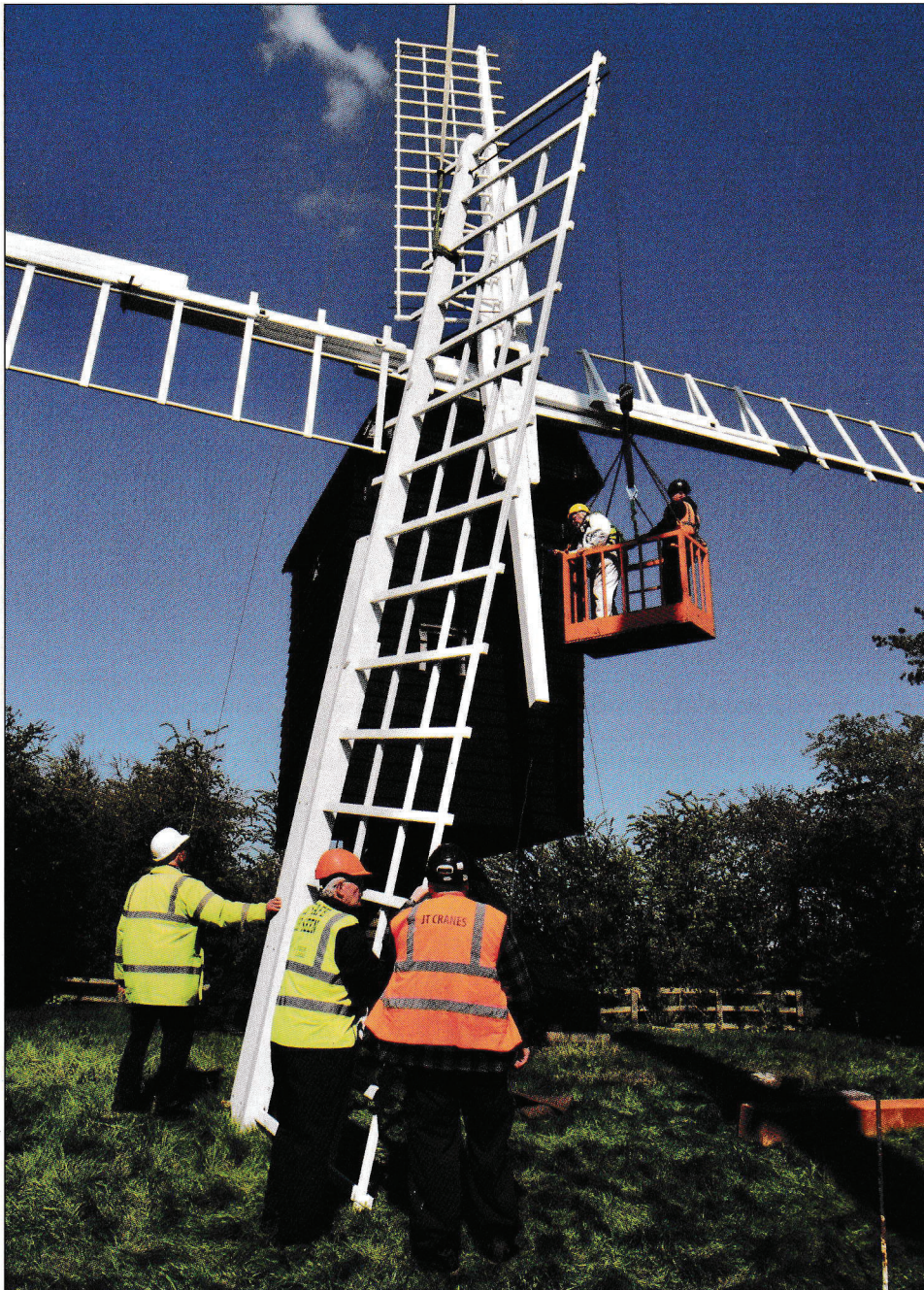
Fitting the last sail to Great Gransden post mill (Cambridgeshire, UK) by Gransden and Wicken millwrights on 19 April of this year (photograph by Alan Rowbotham).
