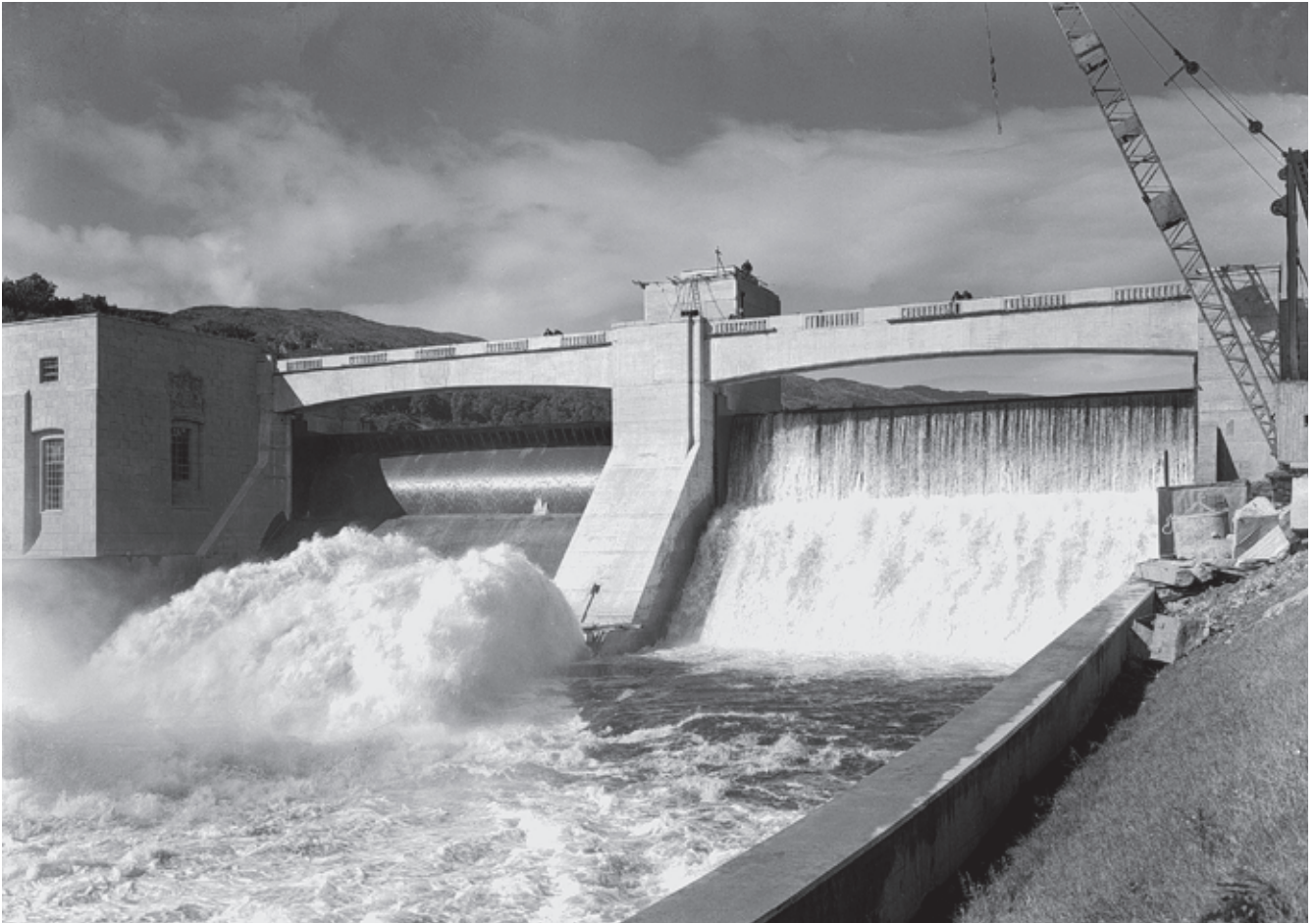
3.7 Pitlochry power station, 1947-1951, Tummel Valley hydroelectric scheme. Crown Copyright: RCAHMS. Licensor www.scran.ac.uk
