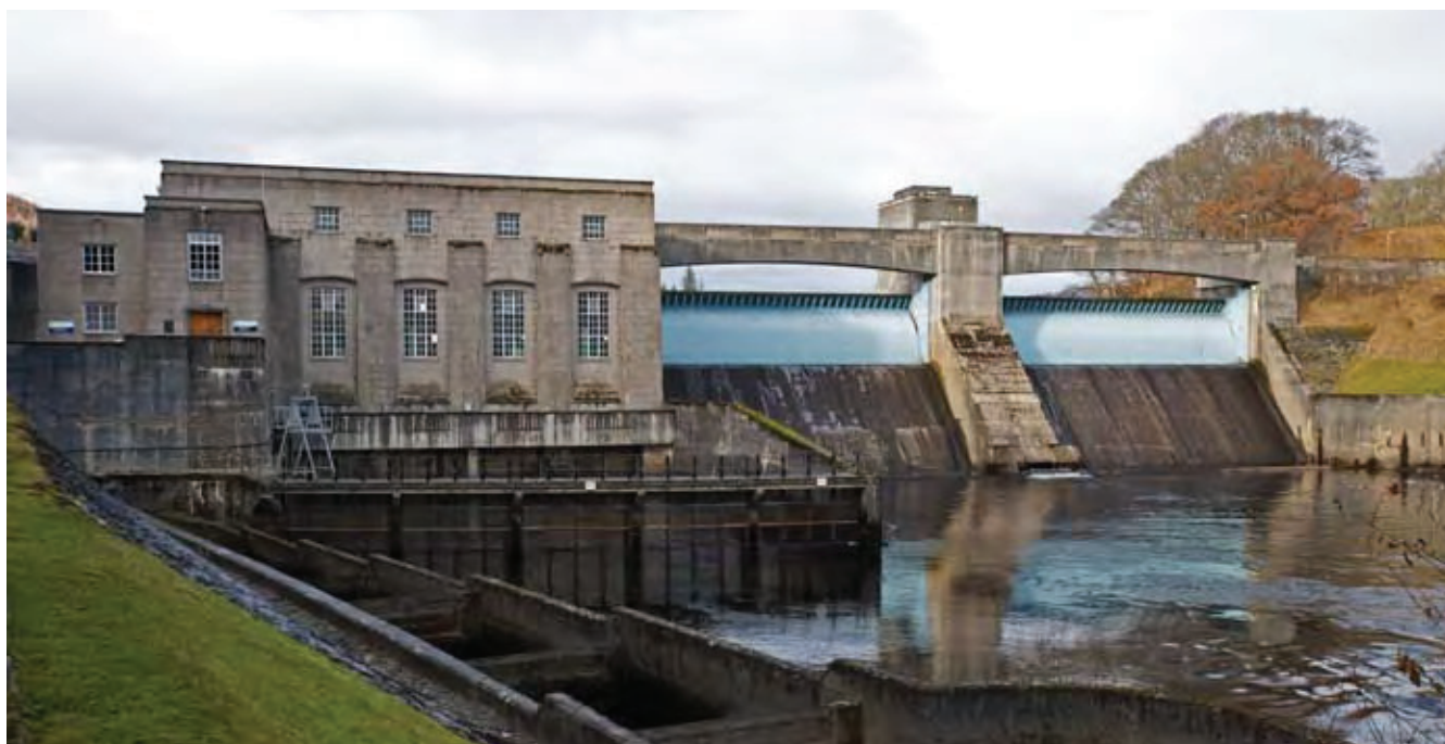
4.6 Pitlochry power station, 1947-1951, Tummel Valley hydroelectric scheme.
