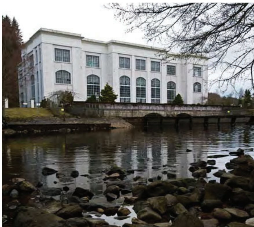
5.1 Tummel Bridge power station, 1931-3, Tummel and Rannoch hydroelectric scheme.
