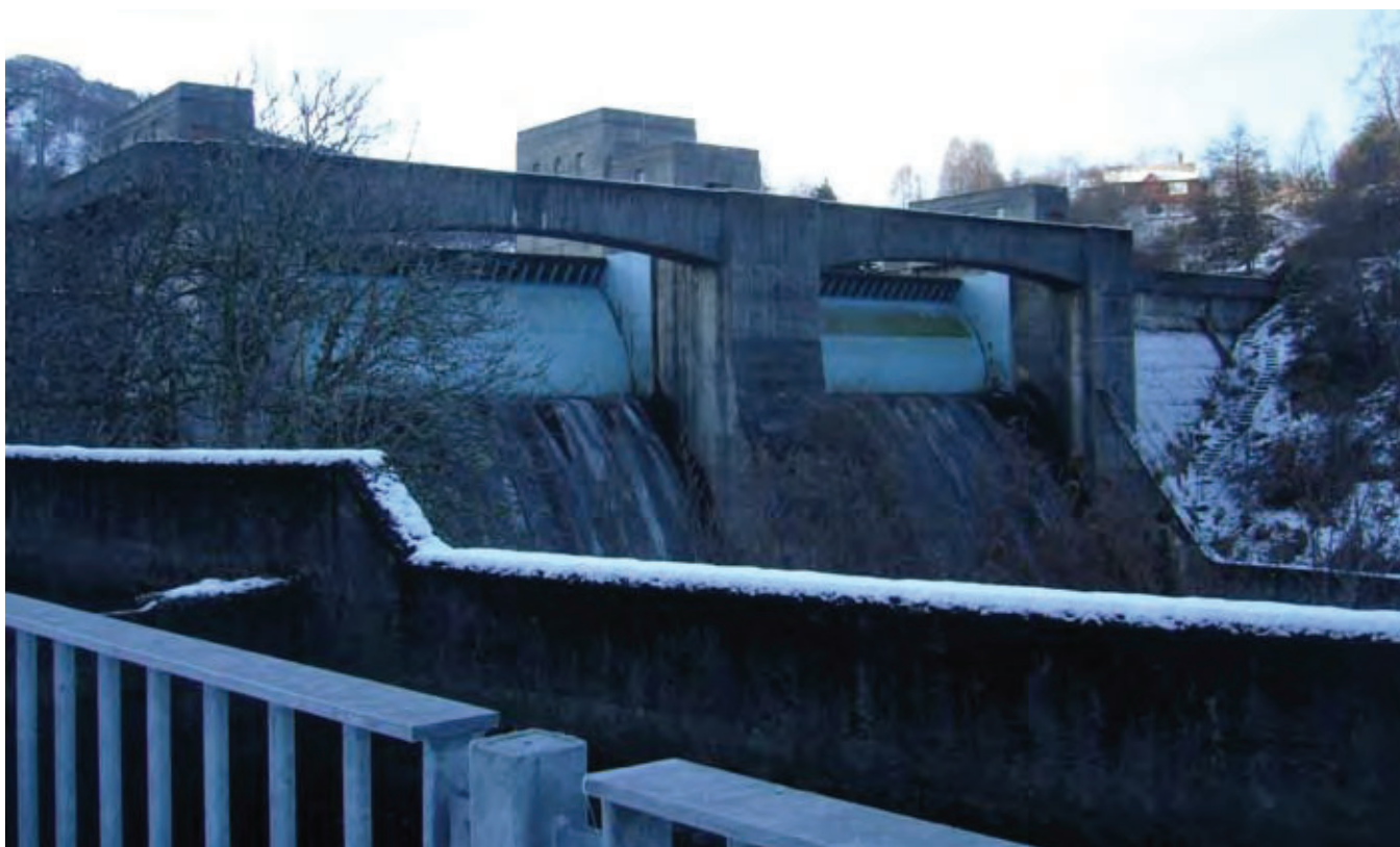
5.8 Clunie dam, 1950, Tummel Valley hydroelectric scheme.
