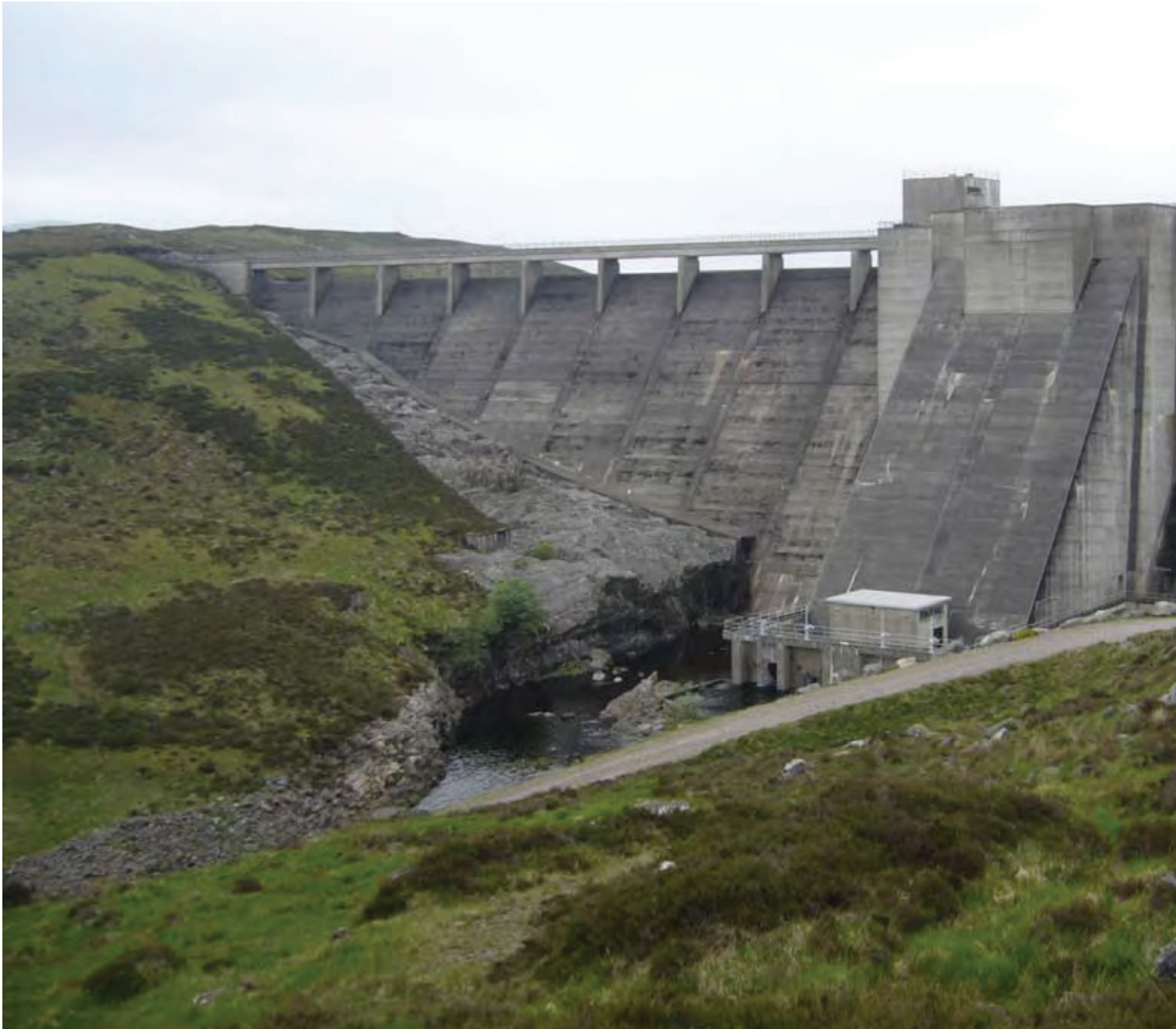
6.7 Orrin dam, 1961, Conon Valley hydroelectric scheme. Orrin dam provides the main water storage for Orrin power station and contains an innovative 4-level fish pass in the large central buttress.
