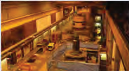
The turbine hall of Cruachan Power Station, buried deep in an excavated cavern beneath the mountain.
