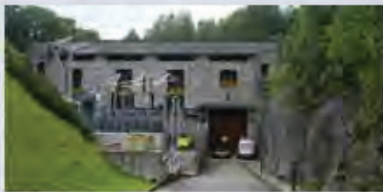
Invergarry power station contains a single high load factor turbine, using water with a low head from the nearby dam.
