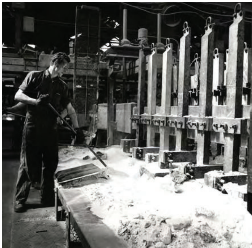
I.3 Aluminium smelting using the Hall-Heroult process, Lochaber smelter and hydroelectric scheme, c.1935. © Glasgow University Archives
