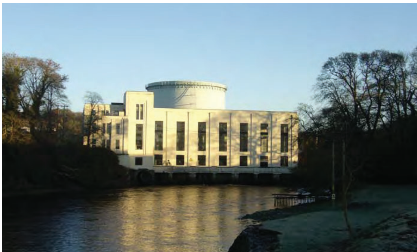
2.6 Tongland power station, 1934, Galloway hydroelectric scheme.
