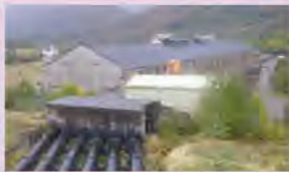
The powerhouse at Kinlochleven with penstocks carrying water through to the turbines inside.
