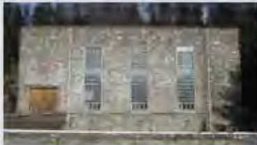
Errochty Power Station, designed by James Shearer and an archetypal example of his use of exposed coursed local stone facings.
