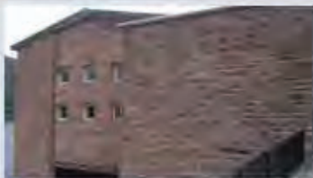
Orrin power station receives water from Orrin dam and is set into a steep bank with a partially buried turbine to maximise the head of water.
