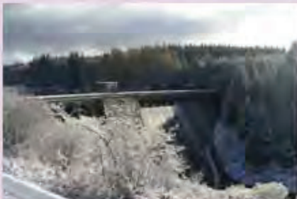
Laggan Dam which provides key storage capacity for the Lochaber scheme.
