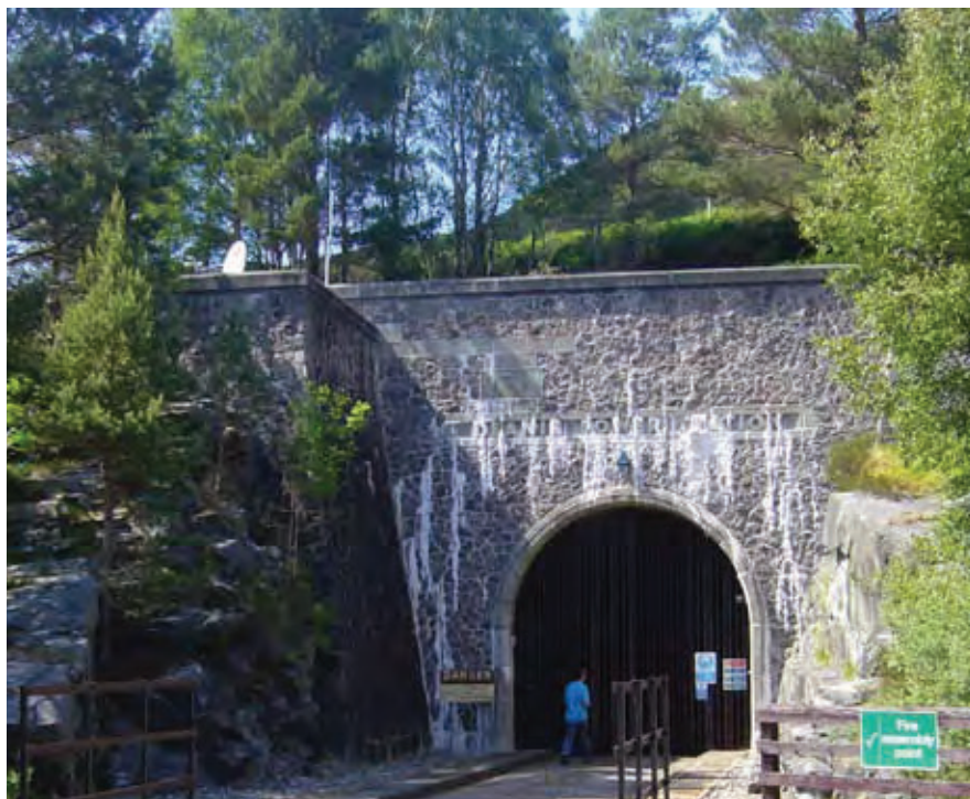
4.2 Deanie power station, 1963, tunnel access portal, Affric hydroelectric scheme.
