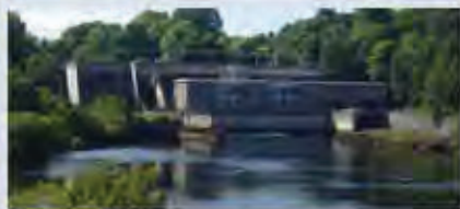
Kilmorack power station is at the bottom of the scheme and is integrated into the dam which regulates the follow of the River Beaully.
