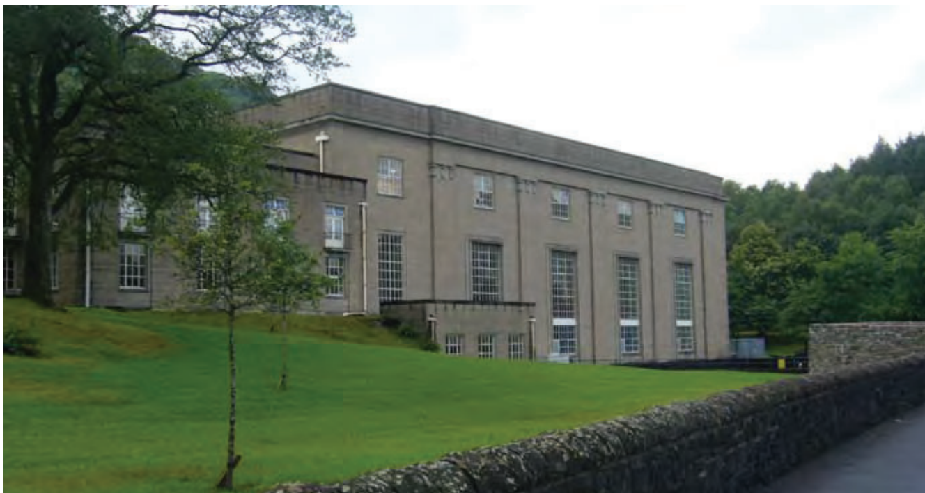
4.3 Sloy power station, 1943-50, Sloy hydroelectric scheme.
