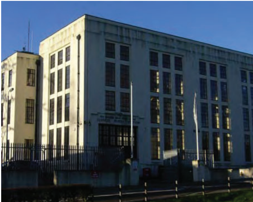
4.4 Glenlee, power station, 1934, Galloway hydroelectric scheme.
