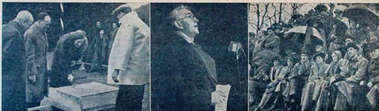
It rained during yesterday's inauguration of the Tummel-Garry scheme at Pitlochry and many of the spectators (right) sheltered under umbrellas. Left, Countess of Airlie lays the foundation stone of the new dam. Centre, Mr Tom Johnston, chairman of the Hydro-Electric Board.
