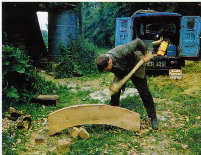
Philip shaping a curb segment with an adze at Stelling Mill in 1968 Picture - Vincent Pargeter
