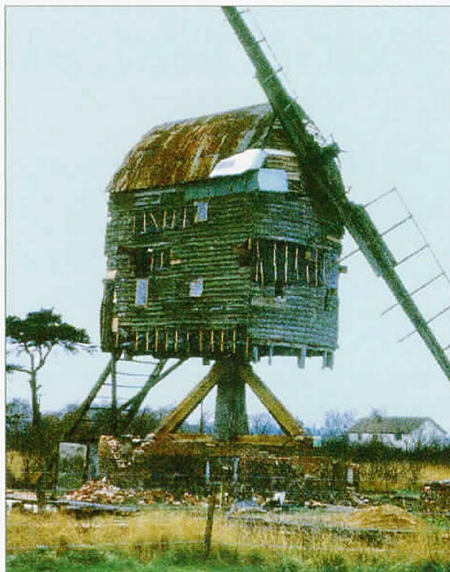
Garboldisham mill 1972 after Philip renewed the wrestle and straightened the buck.. Picture - Vincent Pargeter
