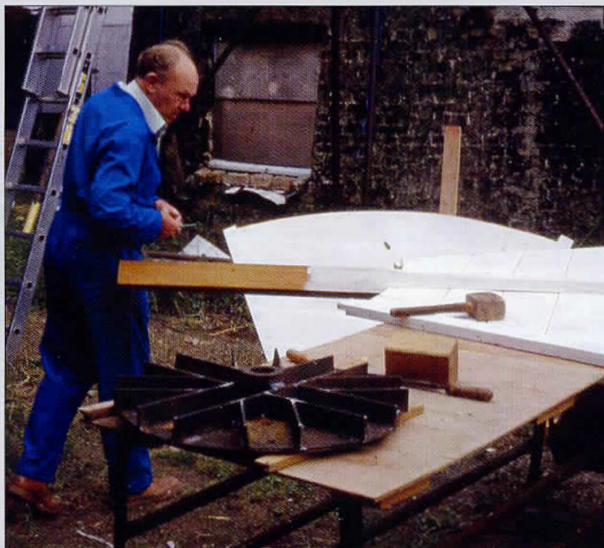
Alan assembling a fantail blade at Wicken in the early 1990s. Picture - Dave Pearce.
