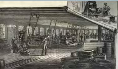
The main site made Gray's famous noiseless roller mills, with the castings and the woodwork for the machines provided by the foundry and woodworking shops of the Reliance Works. For months at a time their daily output reached eight to ten complete machines.
