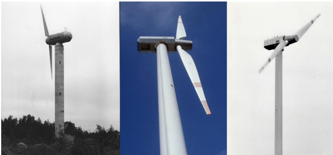
Figure 1. The Kalkugnen and Maglarp turbines. Left: The 60-kW Kalkugnen turbine at Älvkarleby. Photo used with permission from SAAB. Center and right: The 3-MW WTS-3 turbine at Maglarp. Photo used with permission from Jos Beurskens (center, all rights reserved) and Sydkraft/E.ON (right).
