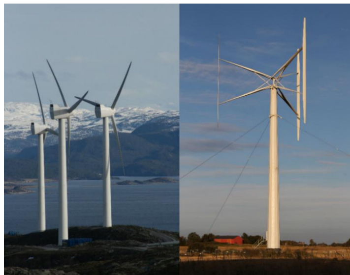
Figure 4. ScanWind and Vertical Wind. Left: ScanWind 3.5-MW turbines at Hundhammerfjellet, Norway. Photo by and used with permission from Anders Wickström. Right: The 200-kW Vertical Wind H-rotor in Falkenberg. Photo by Erik Möllerström.
