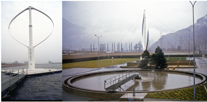
Fig. 3. Left: The 94-kW Pioneer I on its floating platform in Amsterdam, the Netherlands. Right: The 160-kW VAWT in Martigny, Switzerland, with a part of its adjacent biogas system seen in the foreground. Photos by Jos Beurskens. All rights reserved.
