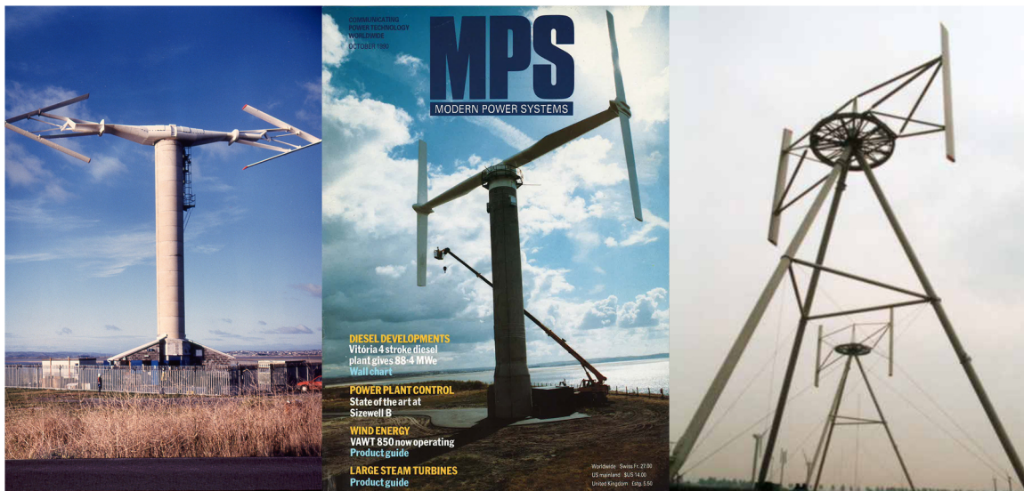
Fig. 4. Left: The 130-kW variable-geometry VAWT-450 with the blades reefered (the blades were straight at maximum power mode). Photo by Jos Beurskens. All rights reserved. Center: The 500-kW VAWT-850 as featured on the front cover of Modern Power Systems in the 1990 October issue. Used with permission from Modern Power Systems. Right: The Heidelberg 300-kW H-rotors in Kaiser-Wilhelm-Koog. Photo by, and used with permission from Jörg Bendfeld.
