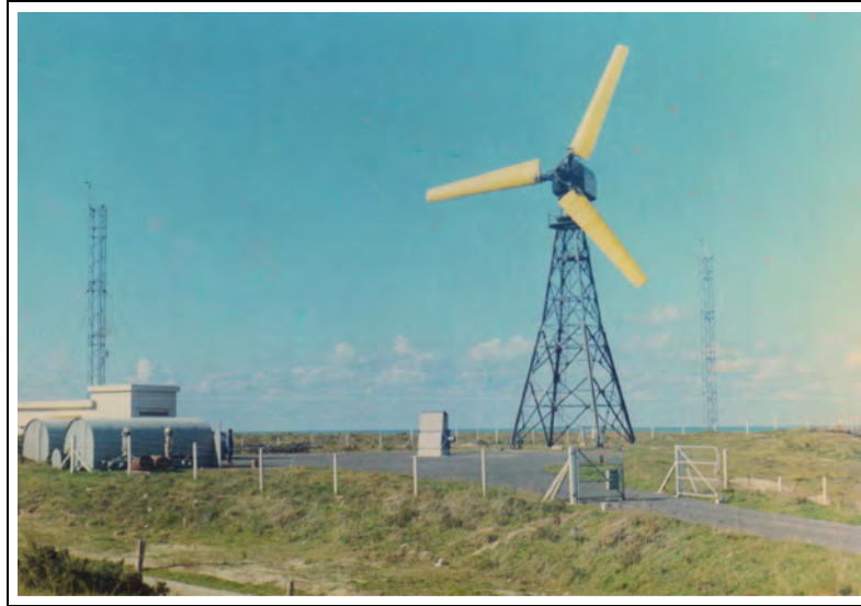
Figure 20. 132 kW Neyrpic. The second iteration of the first prototype in EDF's wind program of the 1960s used composite blades in a rotor 21.2 m in diameter. Of the three turbines in the EDF program, this version was the most successful, generating 700,000 kWh from 1962 to 1966 at a windy site on the Cotentin peninsula. (From the archives of Etienne Rogier).
