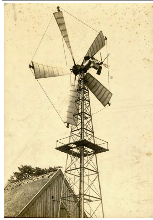
Figure 6. First Interconnected Wind Turbine. The Agrigco was not only one of the first wind turbines to use true airfoils, but also the first wind turbine connected to an AC network. In 1919 a 12.5 m diameter, Agrigco driving a 40 kW asynchronous generator fed AC electricity into the lines of Nordsjællands Elektricitets og Sporvejs Aktieselskab (NESA) at Buddinge north of Copenhagen. Built from 1919 to 1925, the wind turbine use five or six variable-pitch blades upwind of the tower. (The Danish Museum of Energy).
