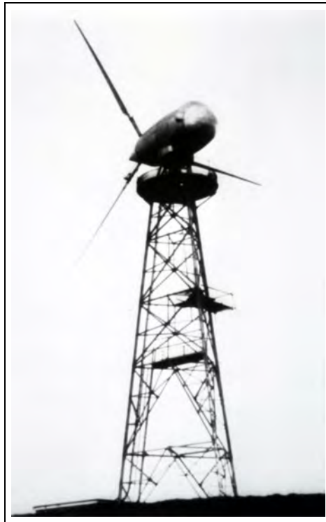
Figure 21. John Brown 100 kW. John Brown Engineering 50-foot (15.24 m) diameter 100 kW downwind experimental turbine at Costa Head, Orkney, Great Britain in 1955. Operated only intermittently connected to the island's diesel network before being removed. (From the archives of Vaughan Nelson via NASA).
