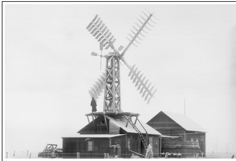
Figure 4. Poul la Cour's klapsejlsmølle . La Cour's original 1891 electricity-generating wind turbine used klapsejls , clap-sails, or jalousie shutters. The self-regulating rotor was 11.6 m (38 ft) in diameter and drove an 18 kW dynamo at ground level. The rotor was oriented into the wind with dual fantails. (Poul la Cour Foundation).
