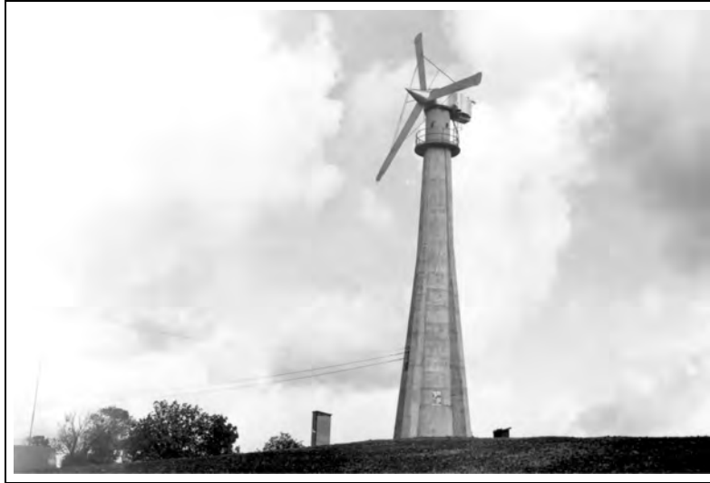
Figure 17. The Mill at Bogø. The forerunner of Juul's Gedser turbine. The Mill at Bogø was 13 m in diameter and drove a 65 kW induction generator. Like his later Gedser design, Juul's Bogø mill used three fixed-pitch blades upwind of the tower with a prominent bowsprit, struts, and stays. (The Danish Museum of Energy).
