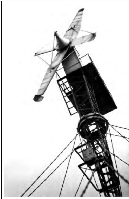
Figure 16. The Mill at Vester Egesborg. Johannes Juul's first attempt at building a wind turbine. The 7.7 m diameter, 15 kW, wind turbine used two fixed-pitch blades upwind of the tower braced with stub blades, struts, and stays, a characteristic seen on later Juul designs. Note the pitchable blade tips. (The Danish Museum of Energy).
