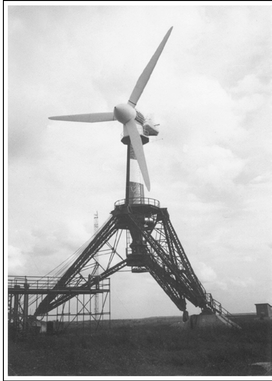
Figure 19. BEST-Romani. The 800 kW BEST wind turbine designed by Lucien Romani. The 30.2 m diameter, fixed-pitch rotor was oriented downwind of the aerodynamically faired, tilt-up tower. The turbine had one of the lowest specific areas (less than unity) of any wind turbine ever built. (From the archives of Jean-Luc Cavey, www.eolienne.cavey.org . All rights reserved.).
