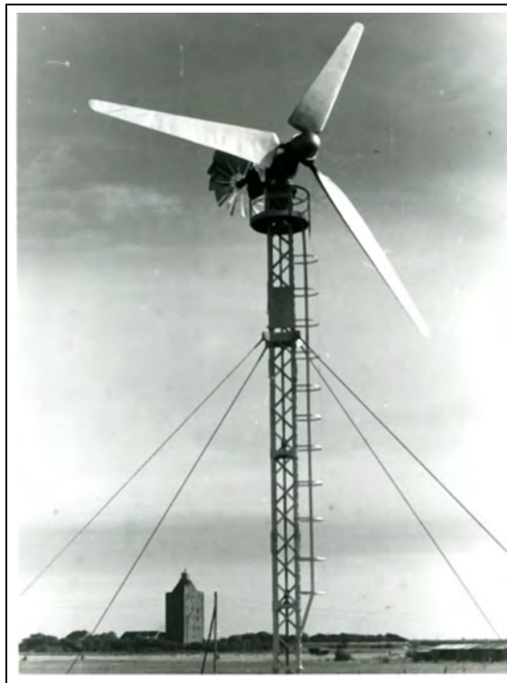
Figure 13. Nordwind 15 m diameter wind turbine on the island of Neuwerk in the Wattensee near the mouth of the Elbe. 1950 Photo by Alfred Ehrhardt. (Alfred Ehrhardt Stiftung).
