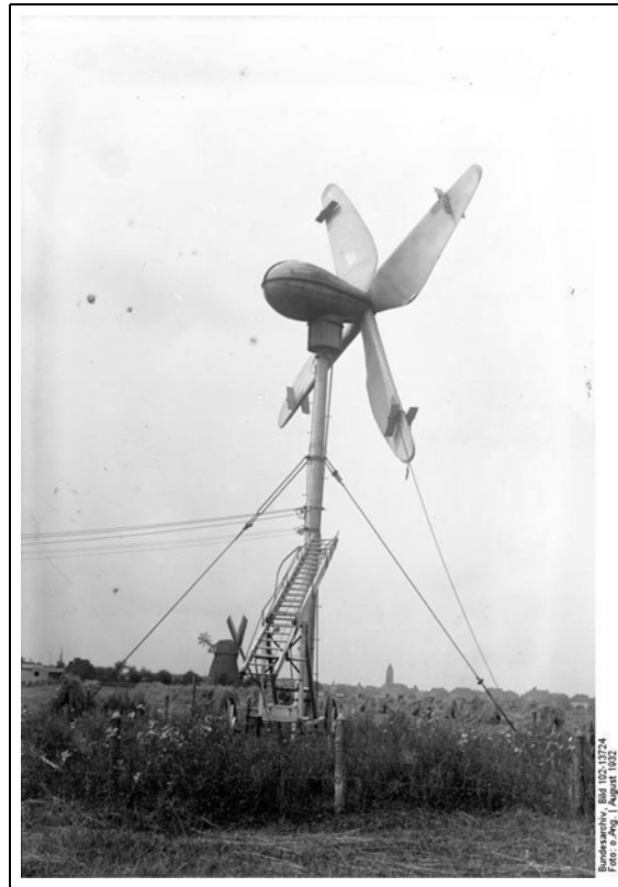
Figure 8. Bilau's Ventimotor. Kurt Bilau's Ventimotor probably at a test field near Berlin in the summer of 1932. The turbine was installed on both a wooden pole and on a steel tube, as shown here. Bilau's turbine was also installed at test field near Oxford in 1925–1926. The rotor is downwind with air brakes and the dynamo was installed inside the stream-lined nacelle. (Bundesarchiv).
