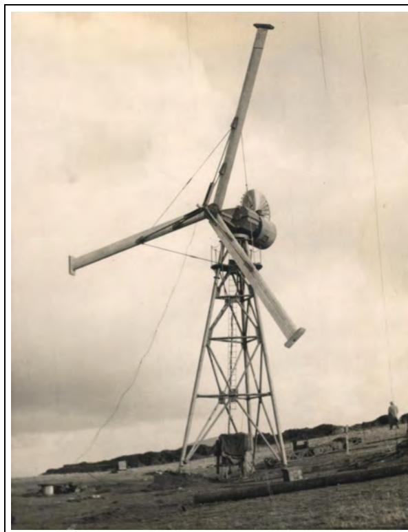
Figure 22. Isle of man prototype. The most successful of the British experiments with wind turbines during the post war period. The 15.2 m wind turbine used a three-blade rotor upwind of the tower, defying a growing convention toward downwind designs. The turbine also controlled overspeed conditions with tip brakes, a feature that wouldn't be seen again for another two decades. (From the archives of Etienne Rogier. All rights reserved.)
