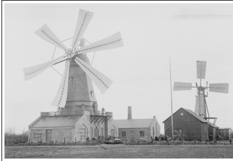
Figure 5. Askov's conical wind catcher. In 1897, Poul la Cour added a keglevindfang or "conical wind catcher" (left) atop Askov's new laboratory. (His earlier turbine is in the background.) The wind catcher used an unconventional six-blade rotor developed by a local millwright. The rotor represented the intuitive thinking of the day, but proved unsatisfactory, leading la Cour to his famous wind tunnel experiments on wind turbine rotors. Eventually, the wind catcher rotor was replaced with a more conventional four-blade rotor designed by la Cour. (Poul la Cour Foundation).
