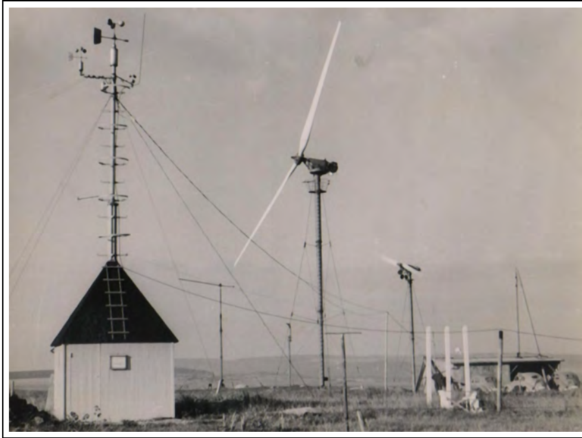
Figure 15. StWG-34 at a test field in the Schwabian Alps. The of climax of Ulrich Hütter's wind turbine development, the StWG-34 was a two-blade downwind experimental wind turbine sweeping nearly 1000 m 2 , and driving a 100 kW induction generator. With a tip-speed ratio of 9.3 it was one of the fastest running of the "fast runners." However, Hütter's ultimate achievement was the development of the attachment of the fiberglass or composite blades to their root flange. Danes would later make the Hütter flange famous. (From the archives of Etienne Rogier).
