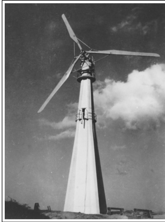
Figure 12. Three-blade F. L. Smidth Aeromotor. Later, larger version of F. L. Smidth Aeromotor installed at Skagen, the northernmost tip of the Jutland peninsula. The three-blade rotor was 24 m (79 feet) in diameter—nearly twice the size of the two-blade turbine—and was braced with struts and stays, a characteristic of later Danish wind turbines. This unit generated nearly 120,000 kWh in 1944, a remarkable performance for wind turbines of this period. (The FLS-files in Danmarks Vindkraftshistoriske Samling).
