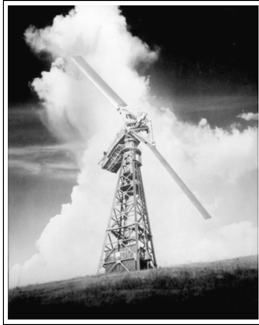
Figure 10. Smith-Putnam. The 1000 kW Smith-Putnam wind turbine used an unusual downwind, flapping two blade rotor 53.3 m diameter. Installed on Grandpa’s Knob in Vermont, it began delivering electricity to Central Vermont Public Service in October 1941. It operated intermittently until it threw a blade on 26 March 1945. It was the first megawatt-scale wind turbine. Machines of this size were not seen again for another three decades. Photo montage by Grant Voaden, Assistant Chief Engineer. (From the archives of Carl Wilcox).
