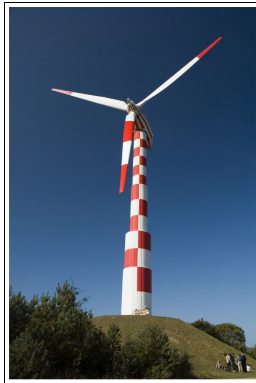
Figure 15. Tvindkraft. World famous megawatt-scale wind turbine installed by students at the Tvind School near Ulfborg on the west coast of Jutland in 1978. Like other pioneering Danish wind turbines, the Tvind turbine is still operating after more than three decades—long after other large turbines installed during the period had been removed and sold for scrap. The turbine's striking pop art paint scheme was created in 1999 by architect Jan Utzon to celebrate the turbine's 25th anniversary. Utzon is the son of the architect who designed the Sydney Opera House.
