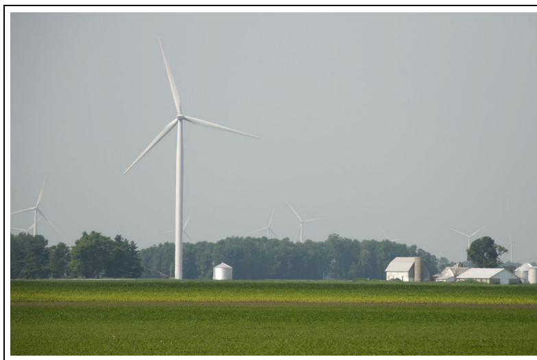
Figure 24. GE 1.6 MW. German utility E.ON installed 125 of GE's 100-m diameter turbines in the first phase of its Wildcat wind farm near Elwood, Indiana. With a specific area of 4.9 m 2 /kW—about twice that of wind turbines manufactured only a decade before—GE's 1.6 MW wind turbine has been designed for areas with low to moderate wind speeds. 2013.
