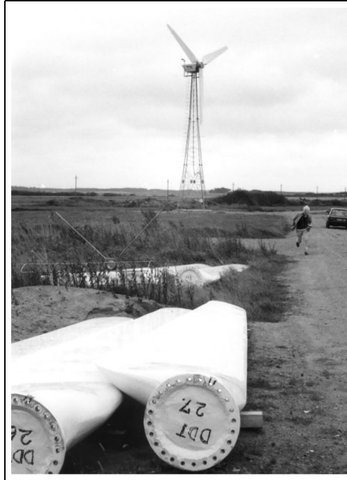
Figure 18. Vestas wind turbine and Økær blades. Background. An HVK wind turbine in Vestas livery at the Vestas plant in Lem. Vestas bought the turbine and design from HVK before launching its successful line of 15-m diameter wind turbines. Foreground. Økær 7.5-m blades with pitchable blade tips developed by pioneering Danish blade designer Erik Grove-Nielsen. Note the “Hütter flange” that made it all work. 1980.
