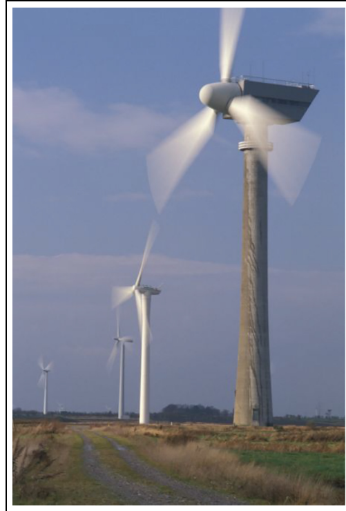
Figure 10. Tjæreborg. The test site at Tjæreborg on the west coast Denmark's Jutland peninsula hosted several megawatt-scale turbines in the late 1990s. The oldest turbine, the 2 MW, 61-m diameter turbine on the concrete tower in the foreground was installed in 1988. After more than a decade of service, it had operated more than 44,000 hours, becoming the longest-running wind turbine in any national or utility-sponsored R&D program worldwide. Note that all the turbines in this photo are in operation, a signature of the Danish program. 1998.
