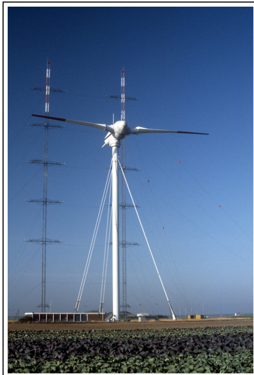
Figure 6. Growian. One of German engineering's most spectacular failures was Growian ( Grosse Wind Energie Anlage ). The downwind, 100-m (330-ft) diameter turbine operated only 400 hours between the time it was installed in 1983 and when it was taken out of service in 1987. Growian operated even less than the Smith-Putnam turbine in Vermont in 1945. It was more than two decades before German manufacturers again ventured to this size. The two guyed towers are meteorological masts at what was to become the Kaiser-Wilhelm-Koog test center. 1987.
