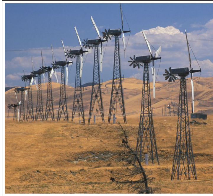
Figure 12. Struts and stays. Like its Danish predecessor at Gedser, the Windmatic 14S (a derivative of Christian Riisager's original turbine) used struts and stays to brace the laminated wood blades. Note the fantail for mechanically orienting the wind turbine into the wind. The blades used pop-up air brakes to limit rotor speed in emergencies. Though ungainly, these wind turbines had operated in California's Altamont Pass for three decades.
