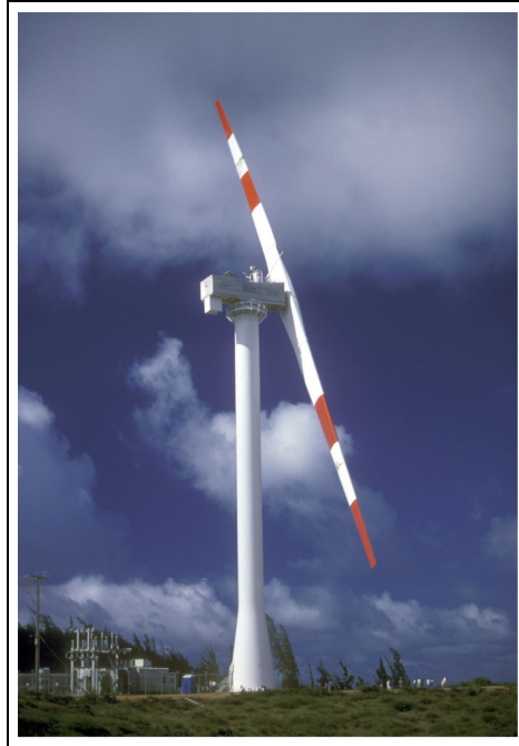
Figure 3. Boeing Mod-5b. The most successful of US DOE's large wind turbines, the Mod-5b marked the end of the line for the program. Though installed nearly one-half decade later, the turbine was as large as Growian with a rotor 98 m (320 ft) in diameter. Unlike Growian, the Mod-5b used a two-blade rotor upwind of the tower, and instead of the fiberglass used in Growian's blades, the Mod-5b used steel. Yes, steel. It was once considered a blade material.
