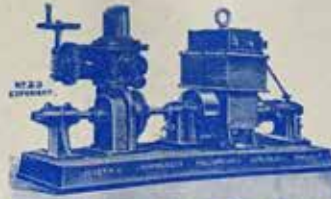
Electric Light Turbine and Dynamo on same Bedplate.
