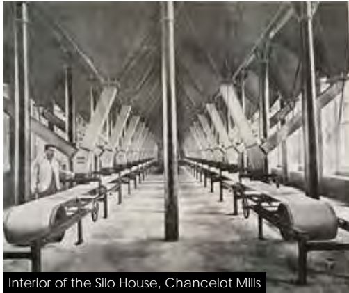
Interior of the Silo House, Chancelot Mills
