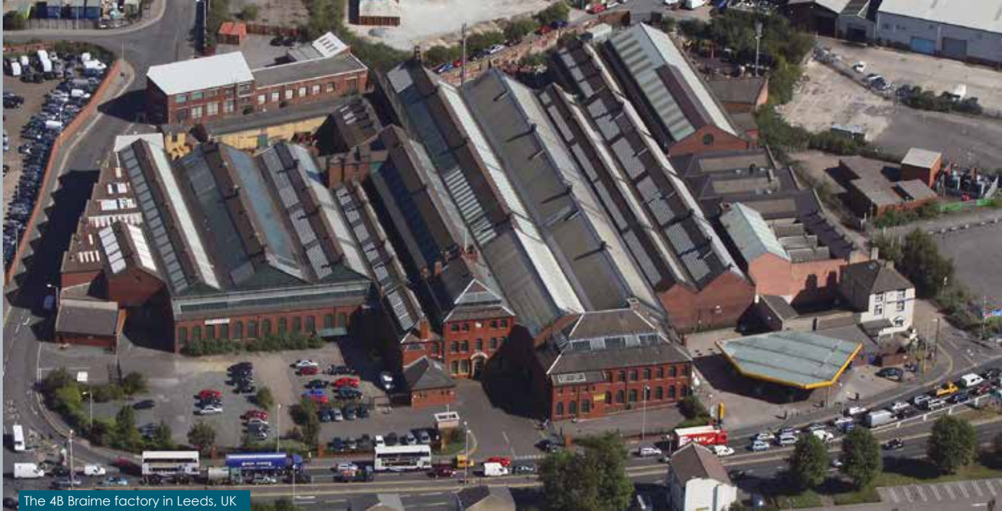
The 4B Braime factory in Leeds, UK
