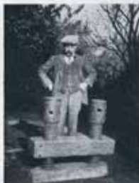
John Russell at Union Mill, Cranbrook, when the sweeps were being restored to the mill. The fantail was made by the millwright.
