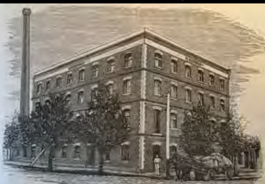
Messrs W Webb and Co's New Roller Mill, Sandhurst
