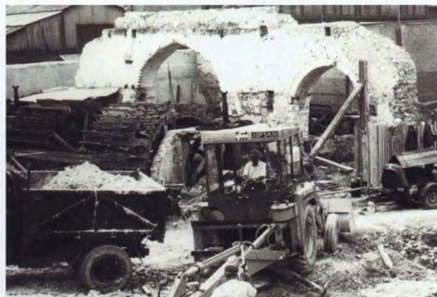
Abbey Mills during demolition in 1964
