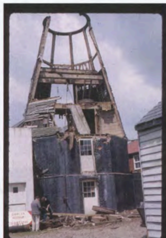
Silverhill windmill being demolished in 1966
